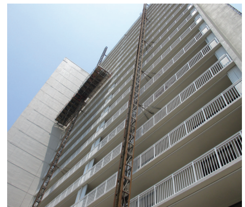
Mast climbers used to access balconies for repairs
