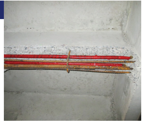
Post-tensioned beam repairs in progress
