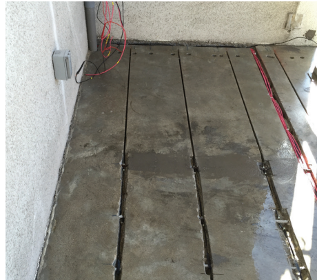
Impressed cathodic protection system installation in progress at balconies
