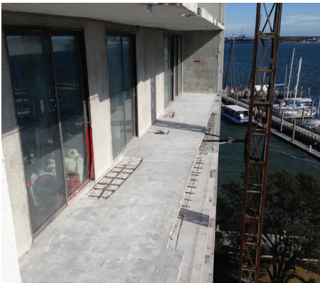
Concrete repairs in progress at balconies
